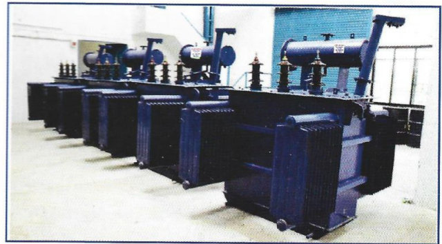
Conservator Type Distribution Transformers
